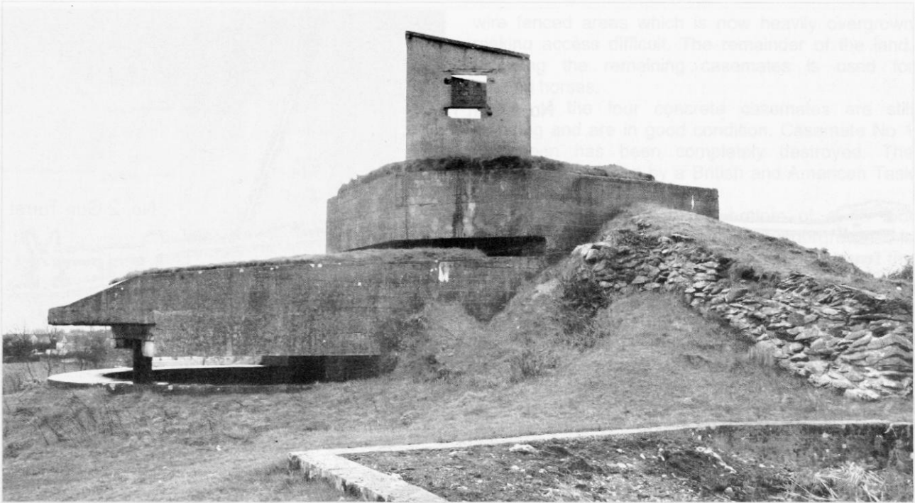
Amfreville - The fire control post at Kriegsmarine Battery at Amfreville
